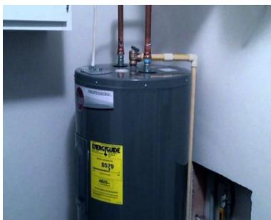
There is nothing better than a hot shower in winter. In the winter months, hot water systems are under an increased load due to the lower ambient temperatures. Is your hot water hot enough? If not, you may need to turn the temperature up slightly. Also, check for any leaks or rust marks around the outside of the hot water tank. Finally check that the safety relief valve is functioning correctly (check your water heater manual for more information).
