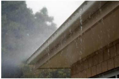
Before the winter rains begin, now is the time to make sure your stormwater drainage pipes, downpipes and gutters are all clear, or you might end up needing to tackle leaks and overflows. Pour a bucket of water into your gutters and downpipes to ensure water is flowing freely. An overloaded gutter can pull away from the house, requiring serious repair costs.
